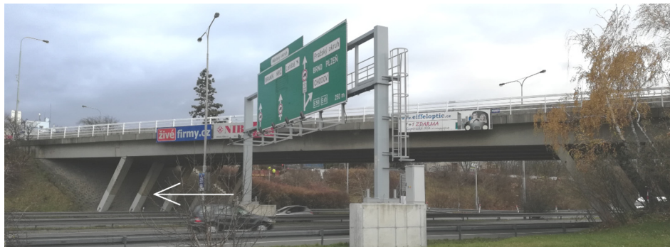
Fig. 11. Bridge view with the analyzed strut.
